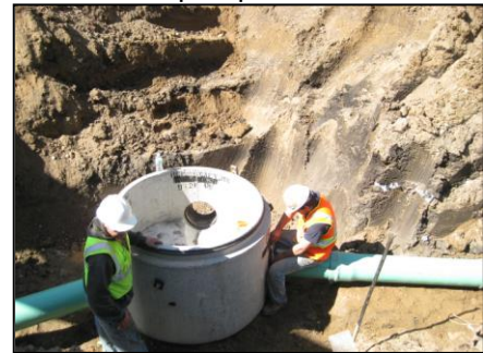
Installation of 48" Manhole Structure – Pump Station 710
