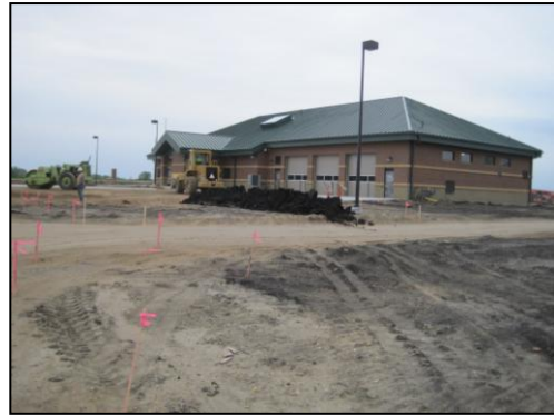
Site and Road Preparation by Admin. Bldg.
