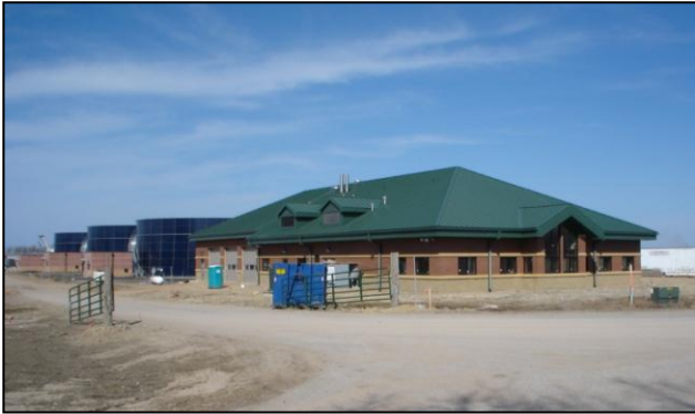
Administration Building and Site Looking to the Northwest
