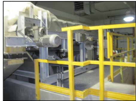
Chemical Room – Secondary Building Structure 250
