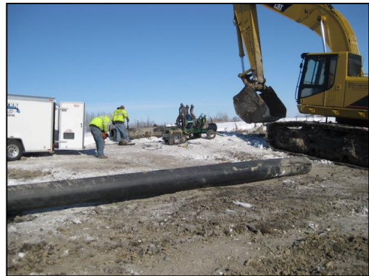
Fusing 16" HDPE Forcemain along CR15
