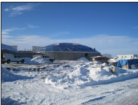
Municipal Clarifier Structure 254
