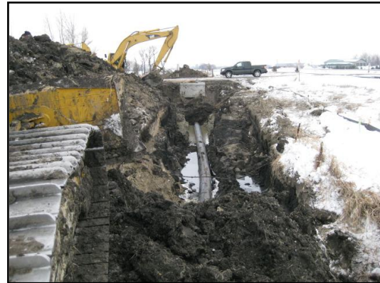
16" Forcemain Installation across Wetland and Installation of Cleanout Structure No. 187
