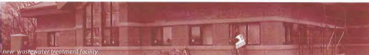
new wastewater treatment facility
