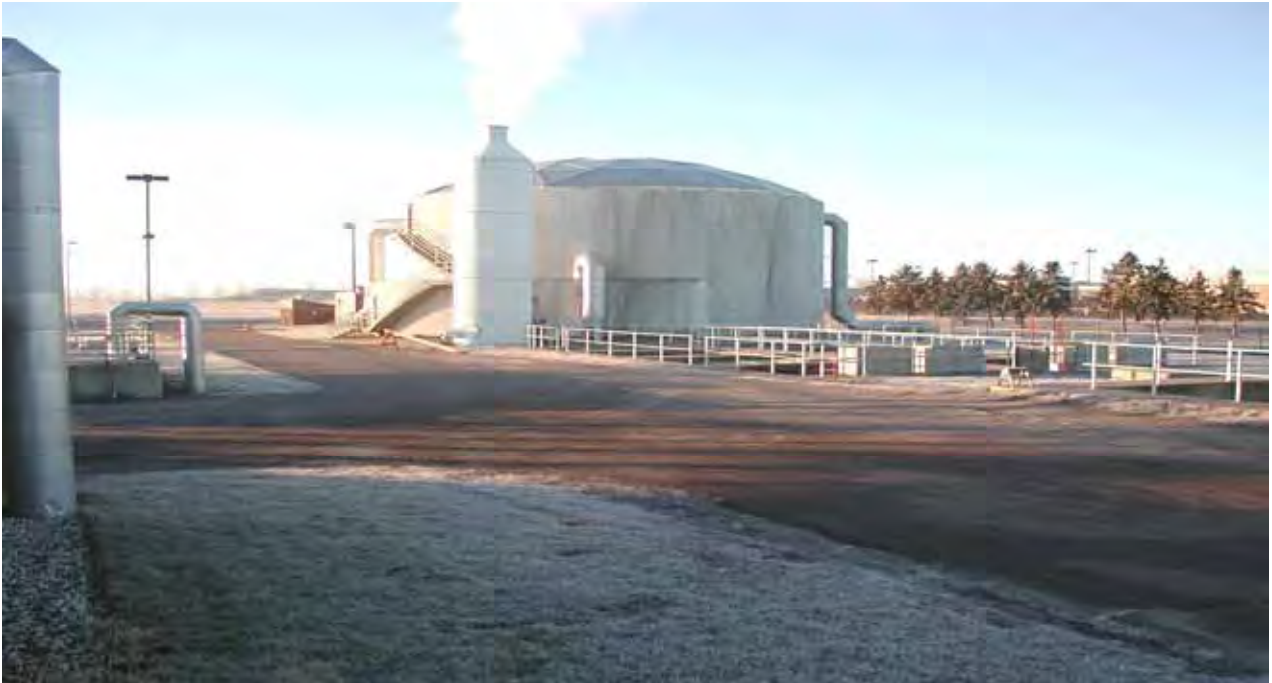
Trickling Filter
