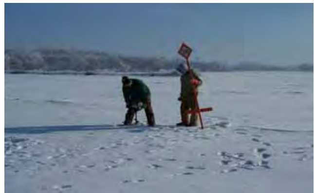
Installing Thin Ice Signs
