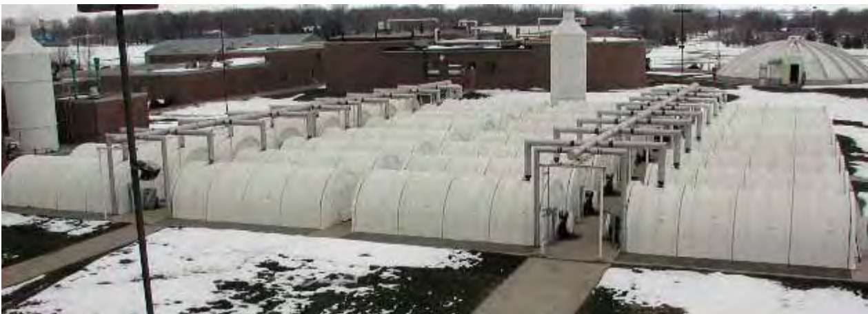
Rotating Biological Contactor's (RBC'S)
