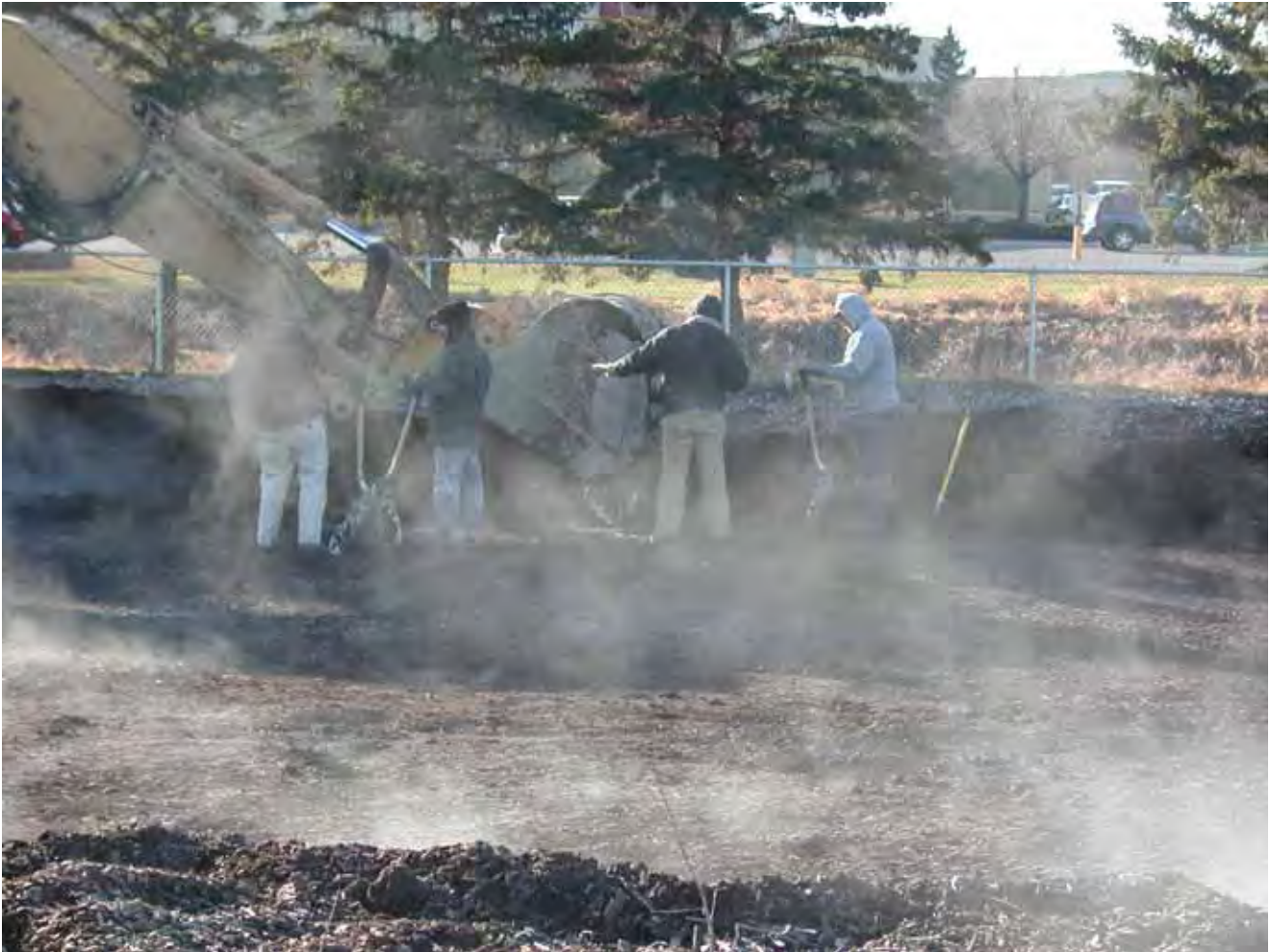
Bio-filter media installation-December 2006
