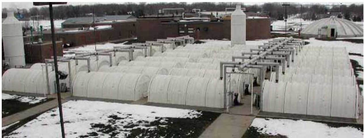
Rotating Biological Contactor's (RBC'S)
